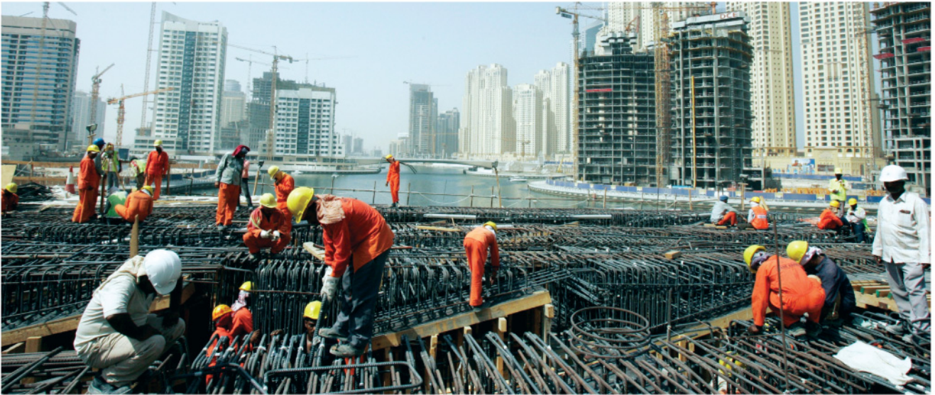
Bangladeshi migrants are working in a construction farm at Dubai
